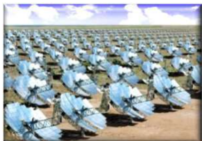
Solar Thermal Farm
