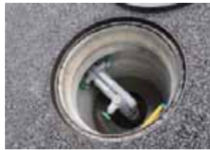
Geothermal heat using pile (Heat exchanger: Borehole)
