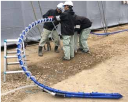
Geothermal heat collecting pile (During construction)
