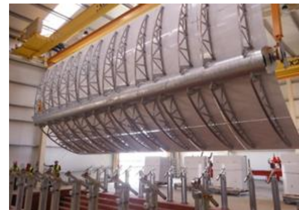
Parabolic Trough Collector Structure assembly line
