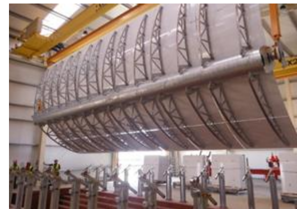
Parabolic Trough Collector Structure assembly line
